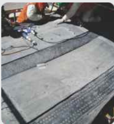
STEELCORD BELT REPAIR
