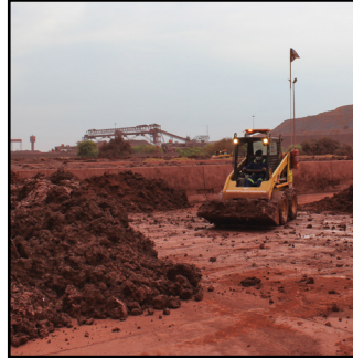
One of GK-IT's mobile bioremediation units in action.
